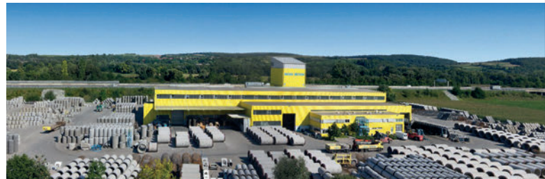
The Haba-Beton site in Nussdorf. Haba-Beton has been running this pipe and manhole production plant near Vienna since 1998.
